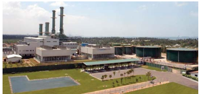
Figure 13. 310 MW combined cycle power plant operating on residual oil.
